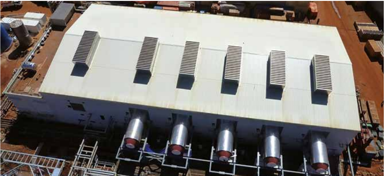
Thika Power Plant - Kenya / Taşyünü Cephe Paneli Rockwool Wall Panel
