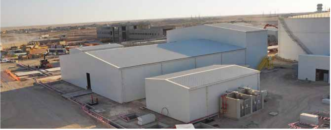
Al Kharirat Power Plant - Irak / Taşyünü Cephe Paneli Rockwool Wall Panel
